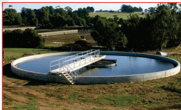
Sedimentation of tank
