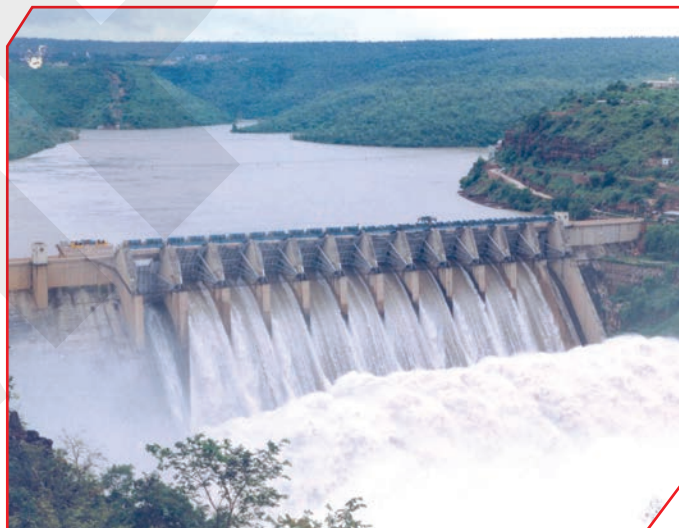
Bhakra Nangal Dam
