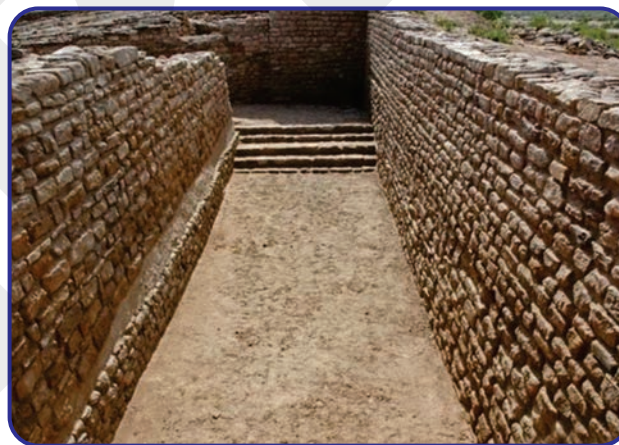
Covered drains along the roads, Mohenjodaro
